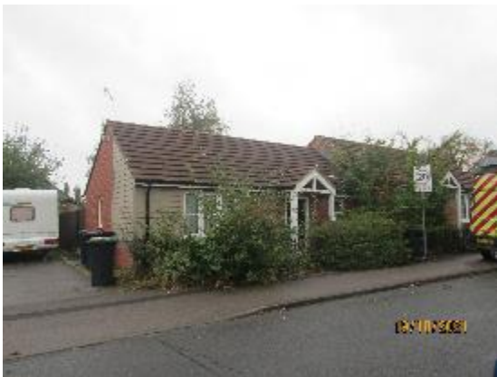
Principal elevation of 8 Midland Road
