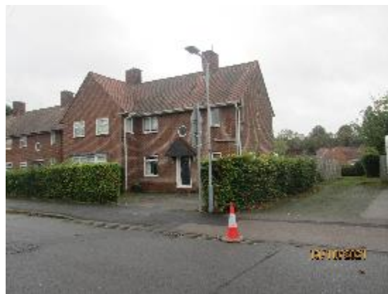
Principal elevation of 10 Midland Road
