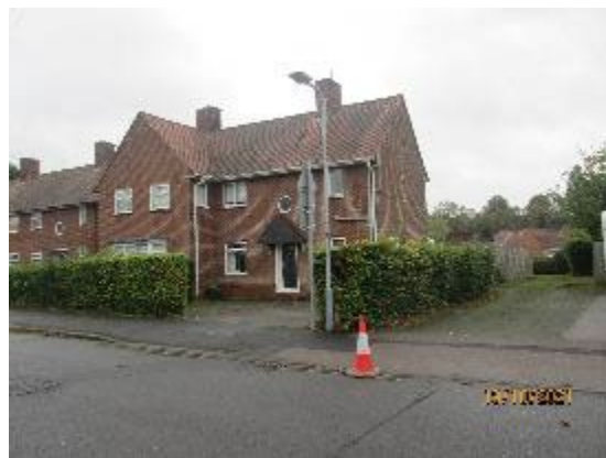
Principal elevation of 10 Midland Road
