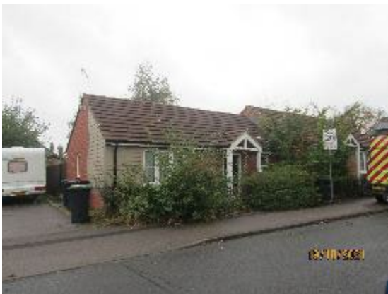
Principal elevation of 8 Midland Road
