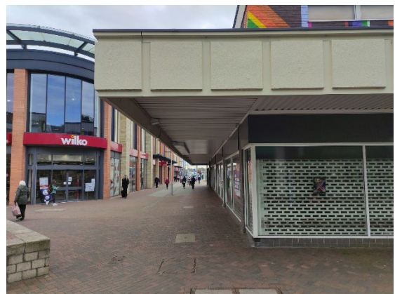
View of existing canopy
